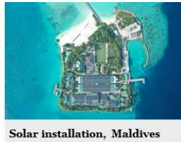
Solar installation, Maldives
